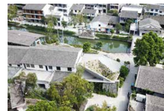
下图：建造中的山根之花鸟瞰；右图：山根之花南立面鸟瞰 Below: the Shangen Flower House under construction; right: aerial view of the Shangen Flower House's southern facade
